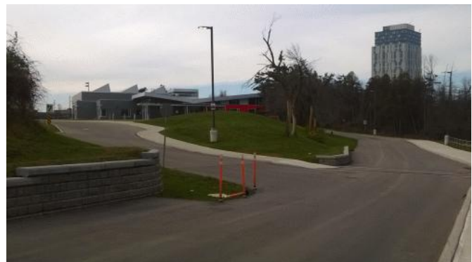
The looong driveway.
